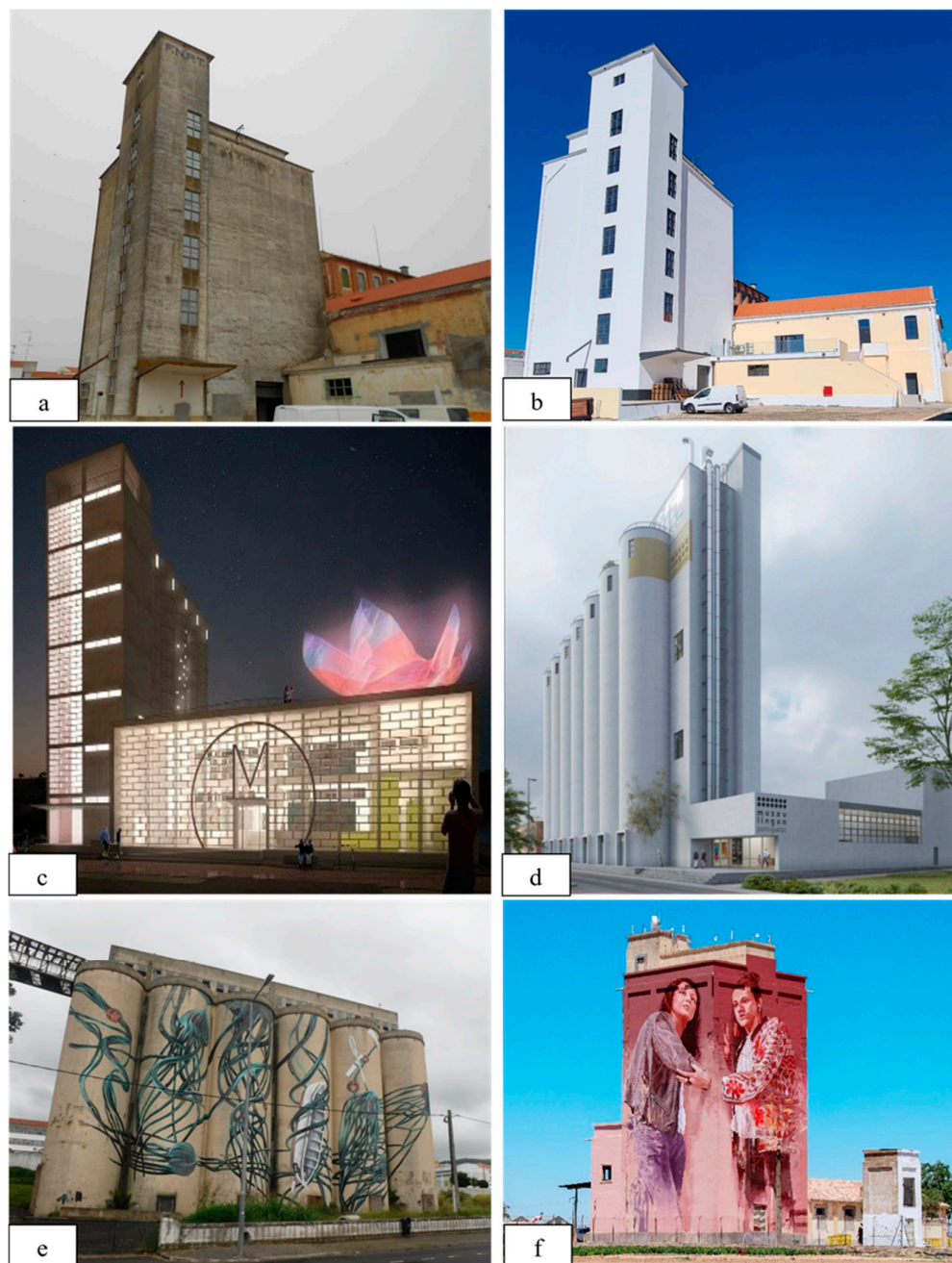
Figure 8. Examples of reused silos. (a,b) Before and after refurbishment of silo in Vila de Boím, Alentejo; (c) 3D view of Museo Zer0 in Catarina da Fonte do Bispo, Algarve; (d) 3D view of future museum in Braganza, North; (e) Silo in Angra do Heroísmo, Isla Terceira, Azores; (f) ‘Titans’ project, silo in Herencia, Spain.
