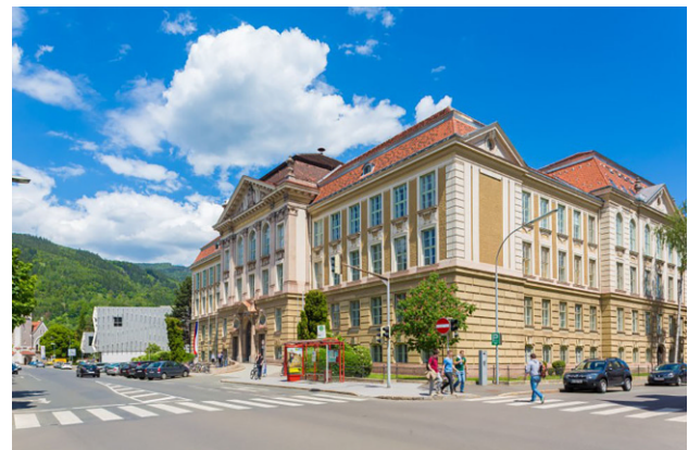
Fig. 1: Main building of Montanuniversität Leoben [2]
