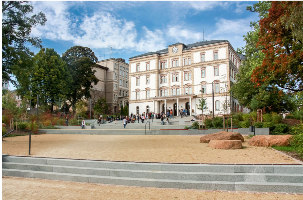
Fig. 6: Main building of Mit-tweida University of Applied Science [10]
