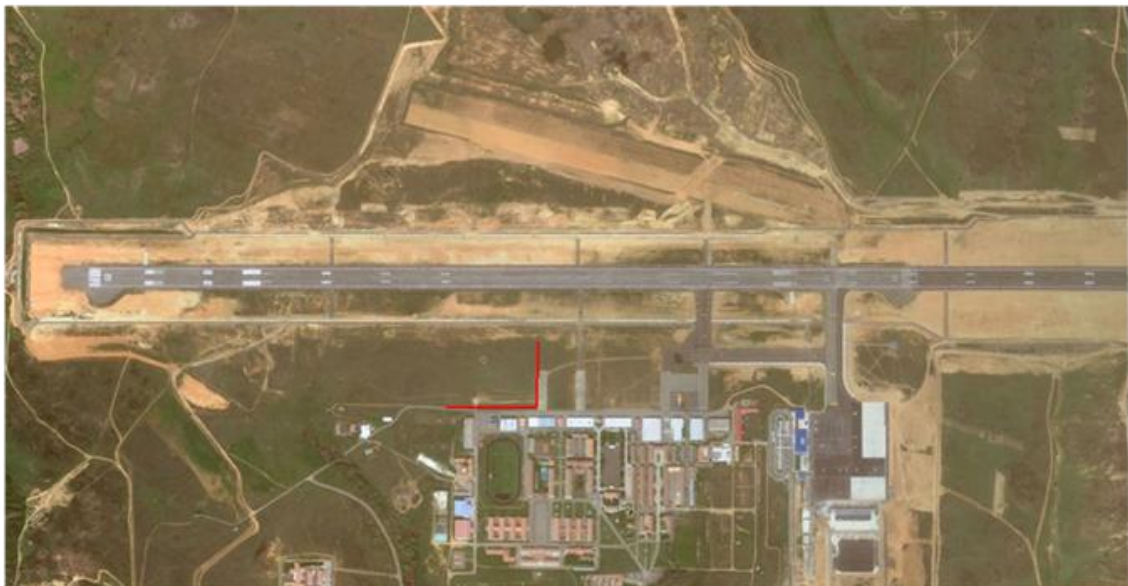
FIGURE 46 WIND PROFILER TEST LOCATION
