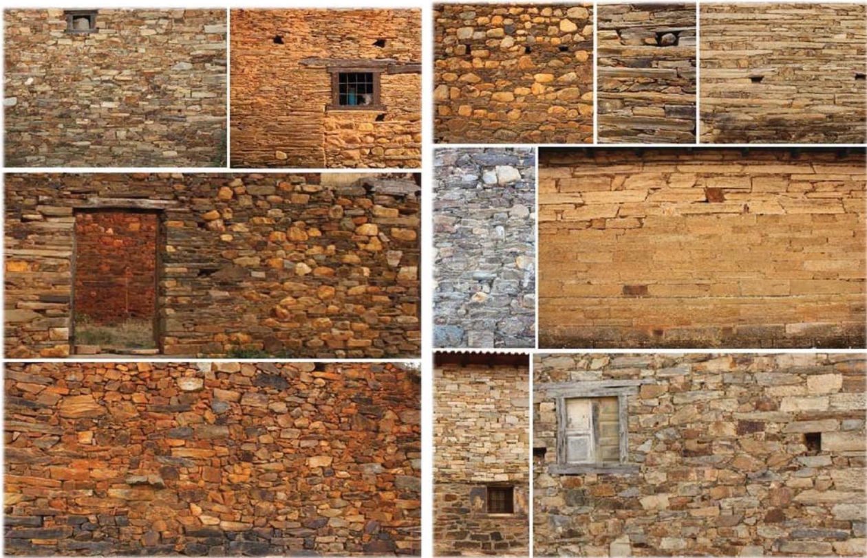
Image 6. A common know-how. Different wall building techniques in Maragatería. Source: Author.
