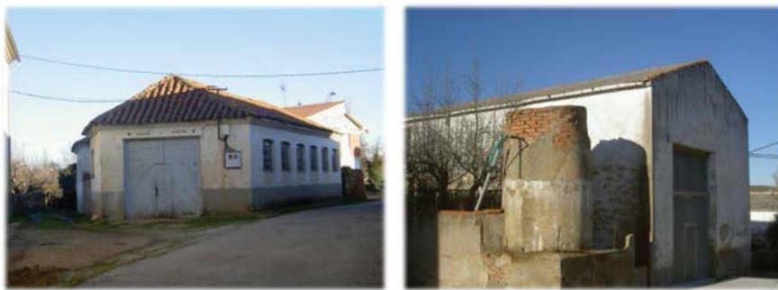
Image 105. Industrial building. Source: Author.
