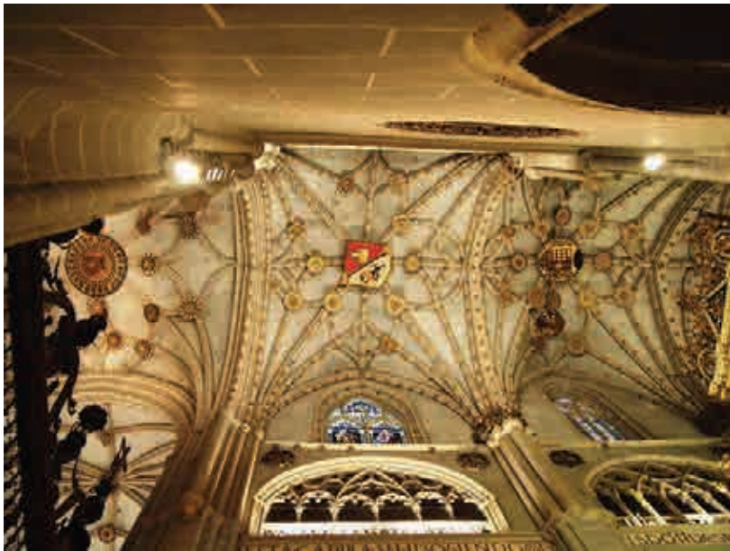
Fig. 11. Palencia Cathedral. Vaults in the aisles and the nave, bay to the east of the transept, with the coat of arms of bishop Pedro de Castilla. Photo by the author.
