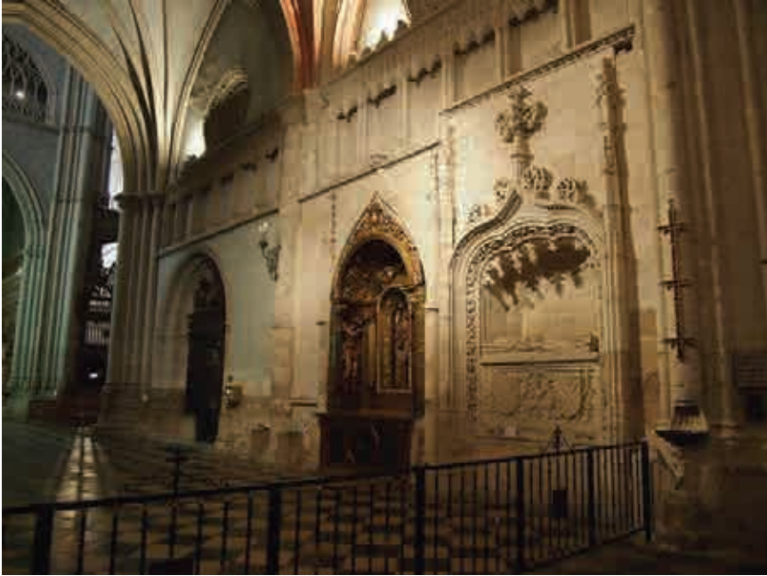
Fig. 9. Palencia Cathedral. Epistle wall of the current high chapel, old choir space. Photo by the author.
