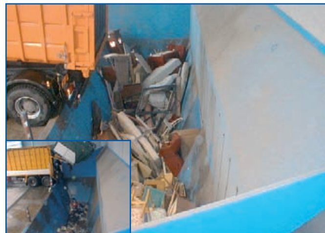
Transfer hopper for 3 parallel dumping places
